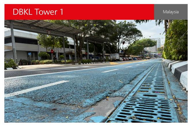
As part of a road improvement project along Jalan Pudu, the government commissioned a drainage upgrade designed to withstand the constant traffic loads from heavy vehicles.
